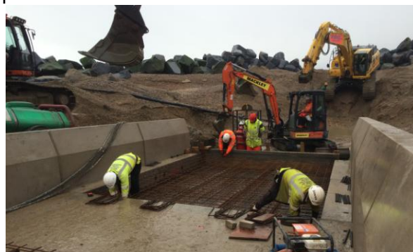
Maintenance ramp toe works on its way
