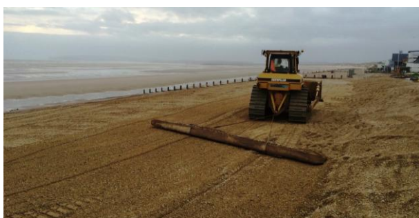
Final levelling works on the recharge
