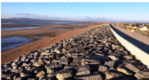
Completed rock revetment and promenade
