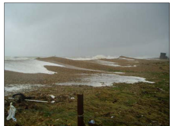
Overtopping at Lydd Ranges
