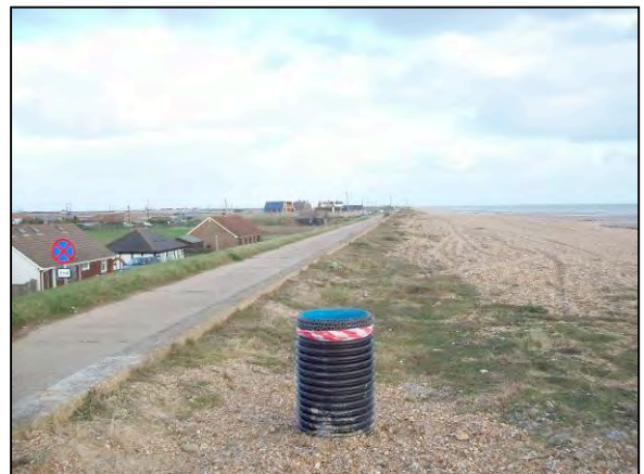
One of the standpipes
