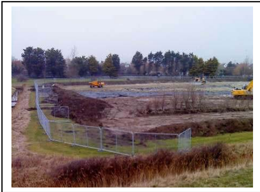
North site compound establishment
