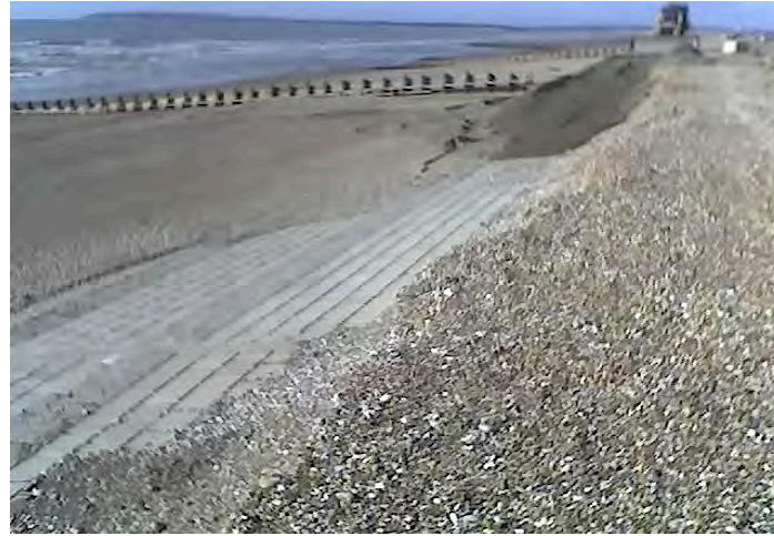
Start of re-shingling at exposed sea wall
