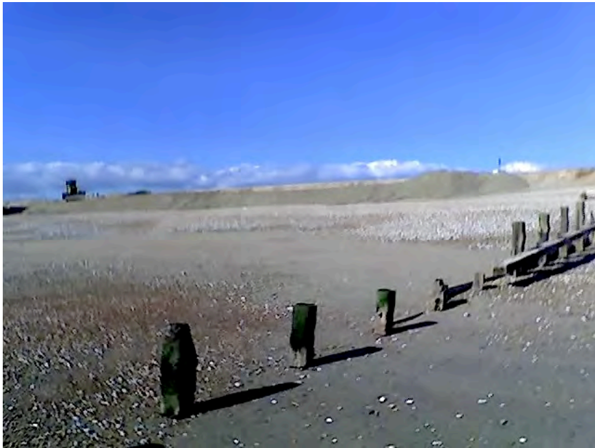
Re-Shingled section covering up exposed old sea wall 9.10.2008 using at least 80 lorry loads of Bretts Shingle
