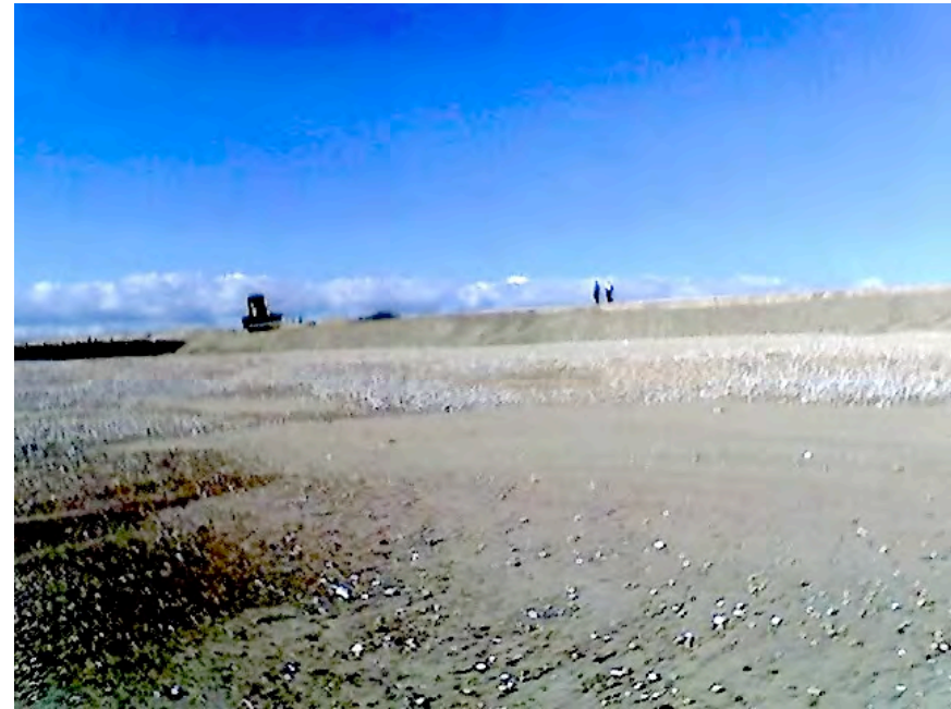
Re-Shingled section covering up exposed old sea wall 9.10.2008 using at least 80 lorry loads of Bretts Shingle
