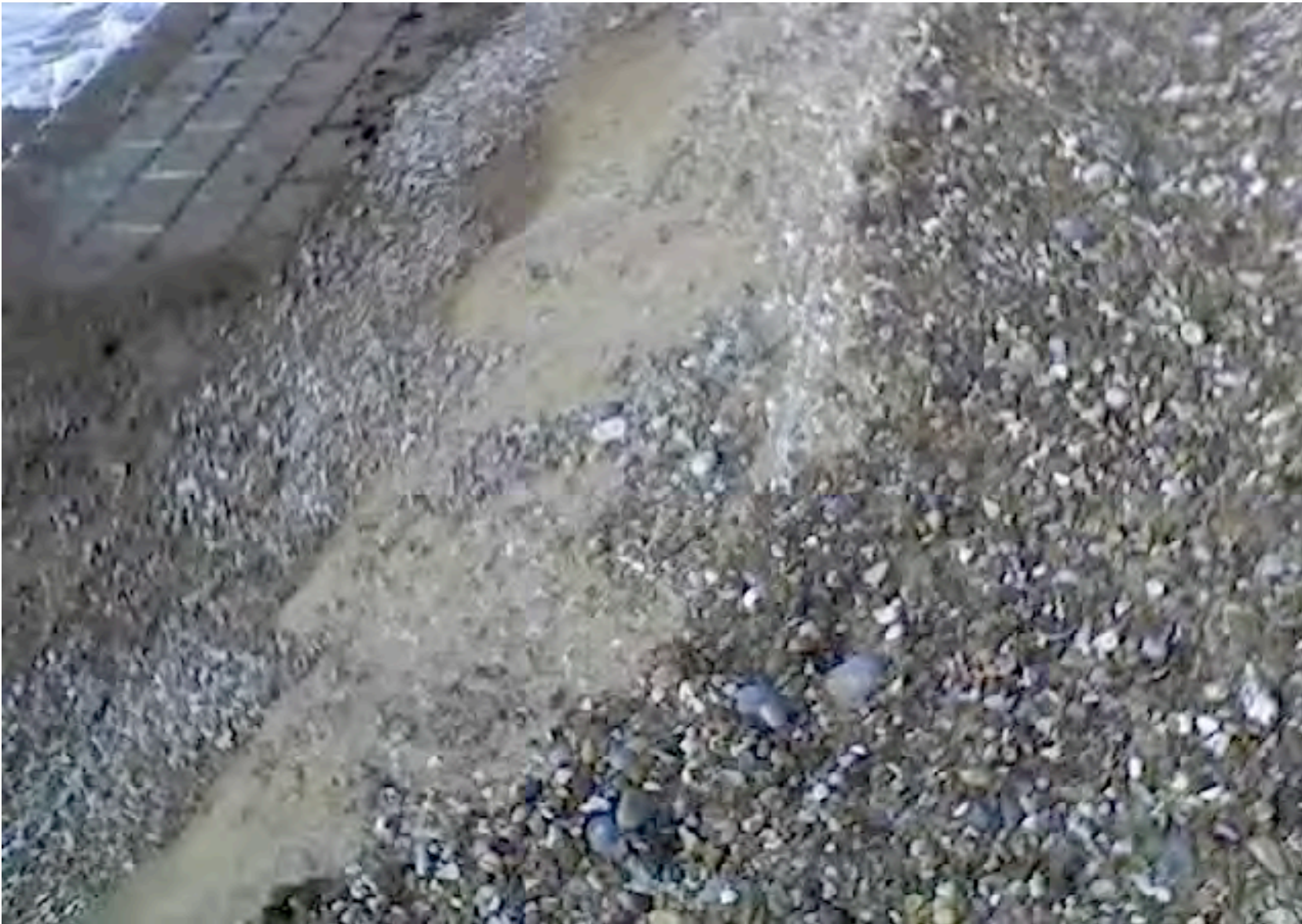
Evidence of sandy material rather than correct shingle quality
