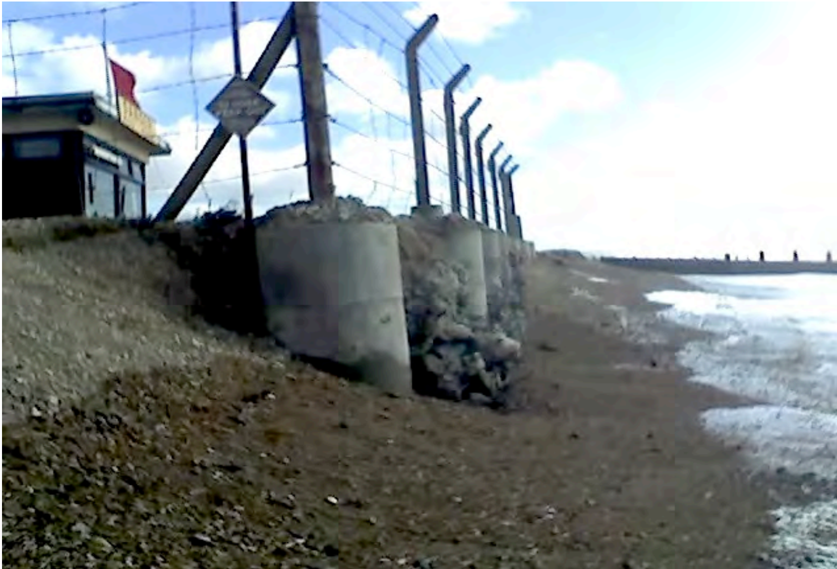
Concrete posts and rock gabions clearly visible
